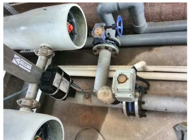
Install of Hydropath
